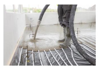
Cemfloor screeds are very responsive to underfloor heating; due to the fact that they can be laid in very thin sections and have a high thermal conductivity of up to 2.9w/mk.
