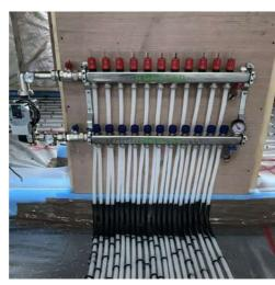
Recommended minimum installation clearances: 200mm between the finished floor level and bottom of the manifold. 100mm above the manifold, 50mm to either side of the manifold and allow an extra100mm for the suply pipe work.
